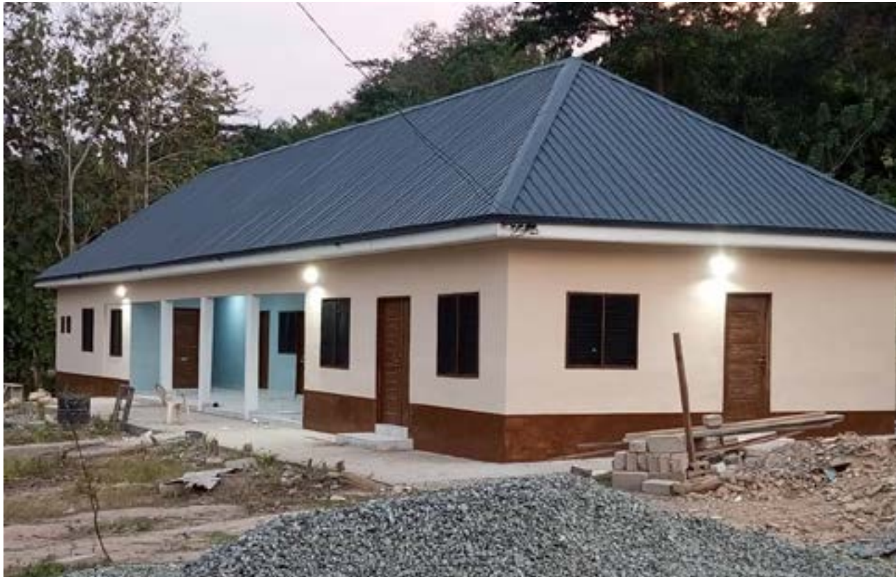
Figure 4.4: Rehabilitation Works on the Leklebi-Kame Health Facility in the Volta Region by the 48 Engineer Regiment of the Ghana Army.
